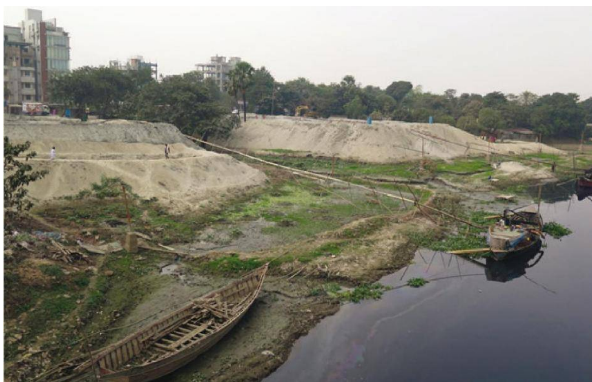
Figure 45 Wetland encroachment for new urban development along Dhaka's ring dike
